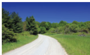
Unpaved Gravel Roads
