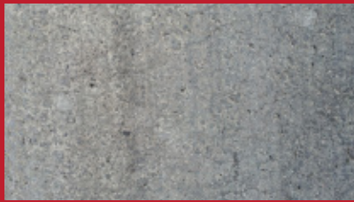
RoadTek-treated road after 7 months of exposure to use and weather
